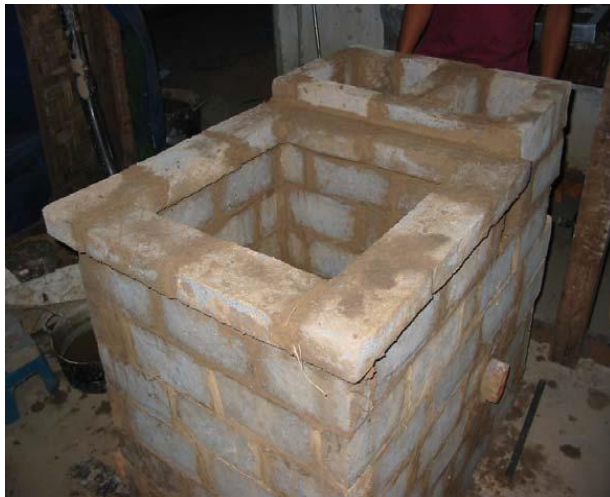
a (foyer en construction)
